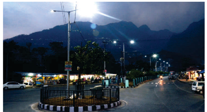
Central Verge on Railway Station Road, Katra with railing and LED lights completed at a cost of Rs. 153 lakh.
